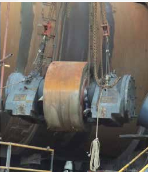
Kiln supporting roller Replacement
