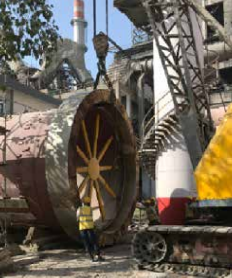
New tire assembly with kiln shell
