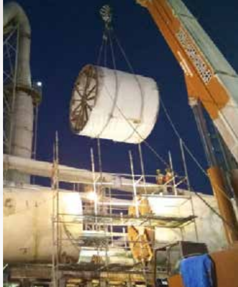
Kiln shell Replacement
