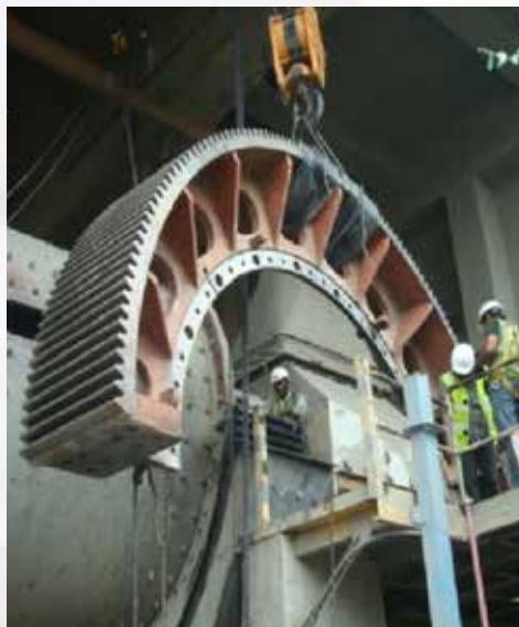
Ball mill Girth gear Replacement
